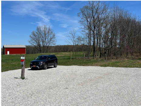
New limestone parking area at trailhead east of SCR 700 East
